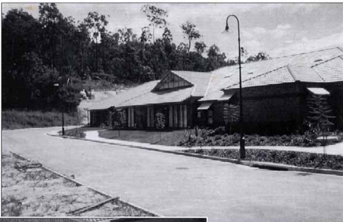
Extensions to Keperra Sanctuary Retirement Village.
